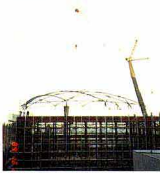
①鋼管7-f建て方
