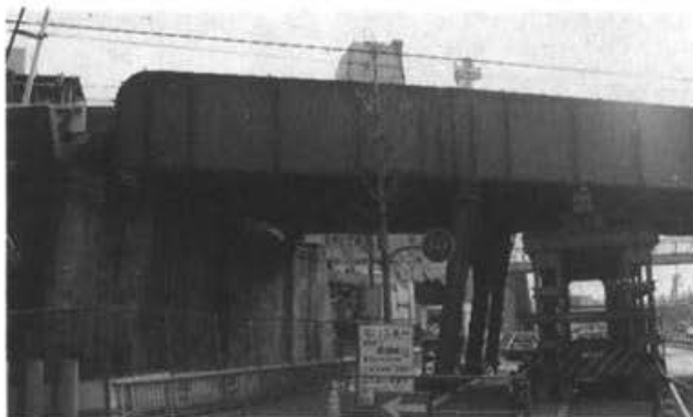
Photo 3.4.11 HANSHIN LINE (Nishi-Nada station)
