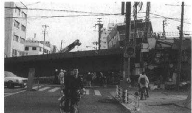
Photo 3.4.8 HANSHIN LINE (Nada-Ward - Oishi-Higashi-cho 5-chome)
