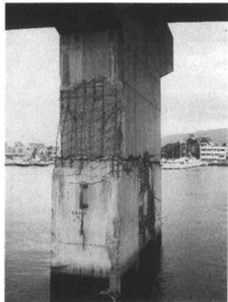
Photo 2.6.3 NISHINOMIYA OHASHI BRIDGE (Nishinomiya-Hama)
