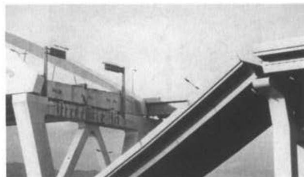
Photo 2.1.13 HANSHIN EXPRESSWAY (Wangan Line )
