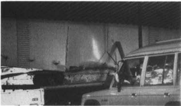
Photo 2.1.3 HANSHIN EXPRESSWAY (Nishinomiya City - Koroen)
