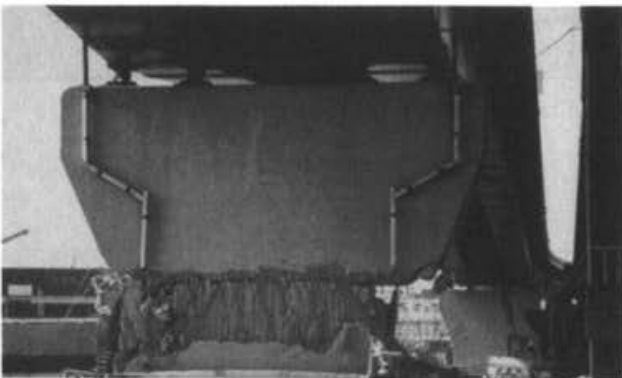
Photo 2.7.1 DAINI MAYA OHASHI BRIDGE
