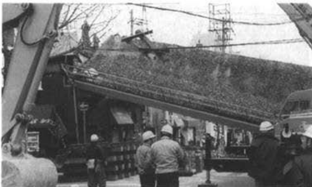
Photo 3.4.7 HANSHIN LINE (Nada-Ward - Oishi-Higashi-cho 3-chome)
