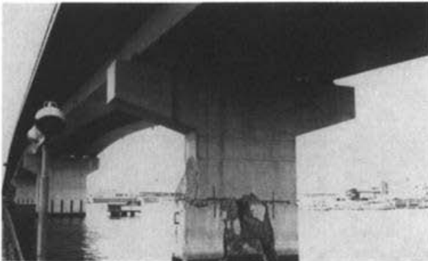
Photo 2.6.2 NISHINOMIYA OHASHI BRIDGE (Nishinomiya-Hama )
