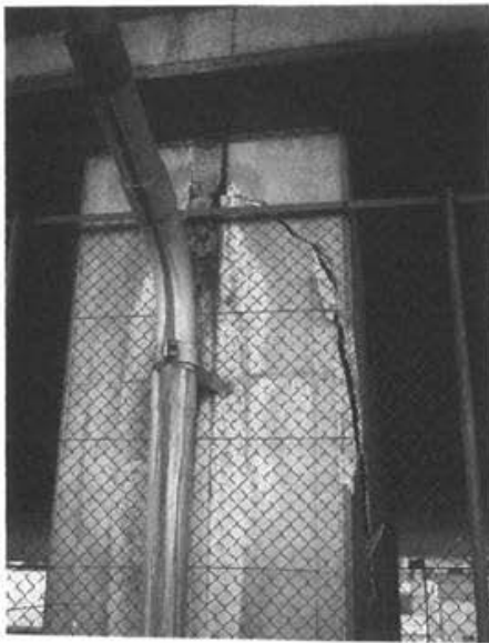
Photo 2.3.3 CHUGOKU HIGHWAY (Itami City - Hagino)
