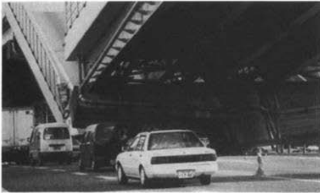
Photo 2.1.1 HANSHIN EXPRESSWAY (Nishinomiya City - Kusugawa-cho)
