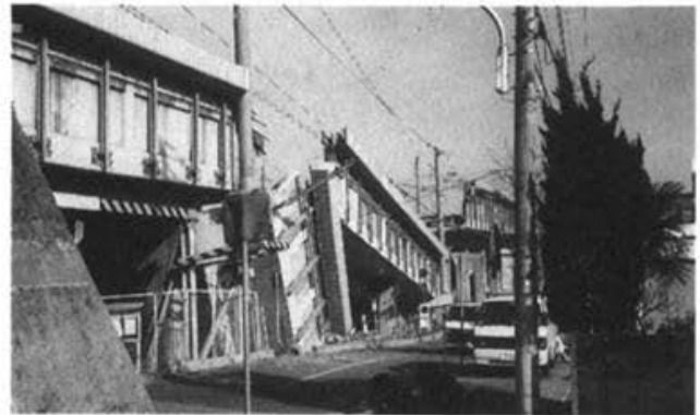
Photo 3.2.8 JR SHINKANSEN (Near Rokko Tunnel)
