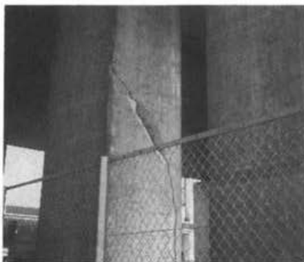
Photo 2.3.1 CHUGOKU HIGHWAY (Itami City - Hagino)
