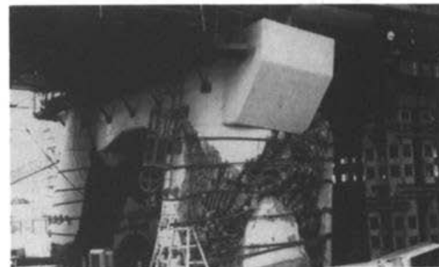
Photo 2.1.12 HANSHIN EXPRESSWAY (Suma-Ward - Ikuhira-cho /JR crossover bridge)
