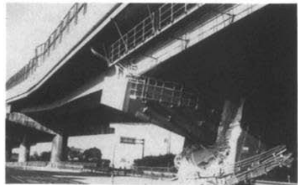
Photo 2.1.4 HANSHIN EXPRESSWAY (Higashinada-Ward - Fukae-Honmachi)
