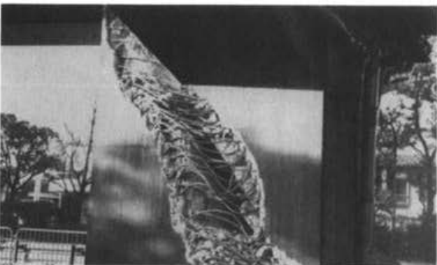
Photo 2.1.7 HANSHIN EXPRESSWAY (Higashinada-Ward - Mikage-Tsuka-cho)
