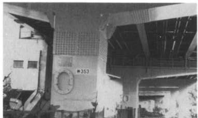
Photo 2.1.8 HANSHIN EXPRESSWAY (Chuo-Ward - Wakihama-cho)
