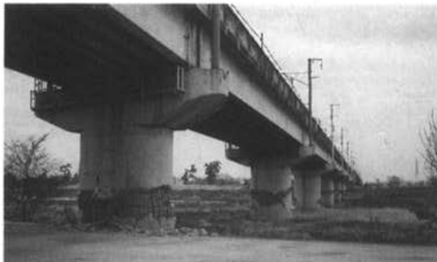
Photo 3.2.3 JR SHINKANSEN (Mukogawa Bridge)
