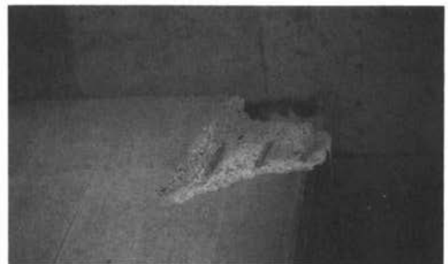
Photo 2.3.2 CHUGOKU HIGHWAY (Itami City - Hagino)
