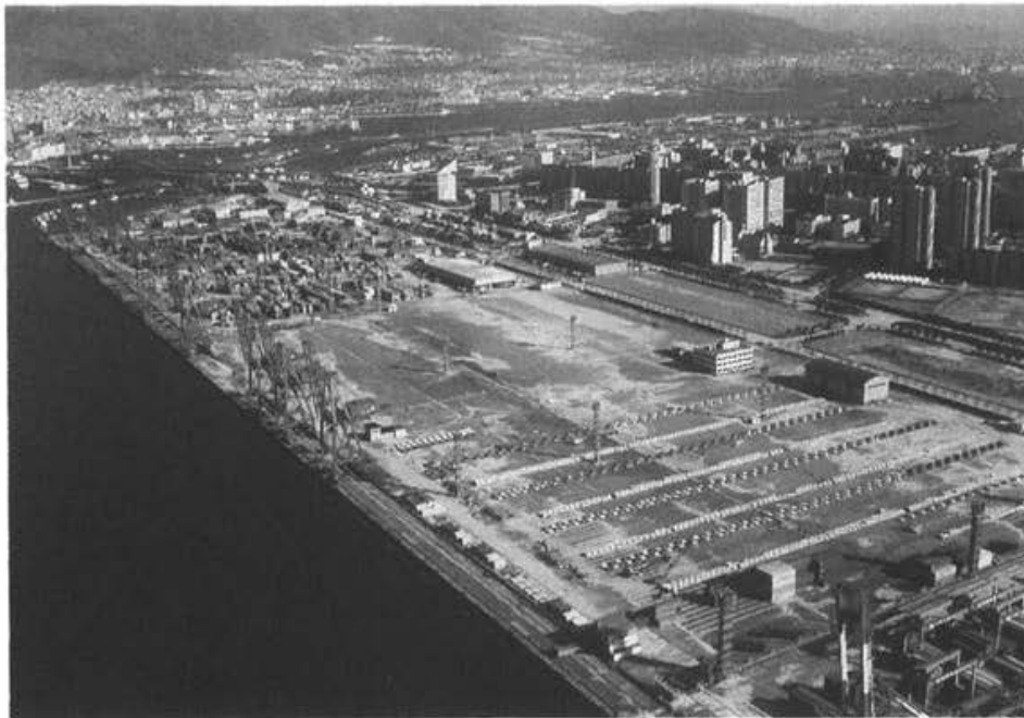
Figure 4 Liquefaction of Container Yard at West of Port Island
