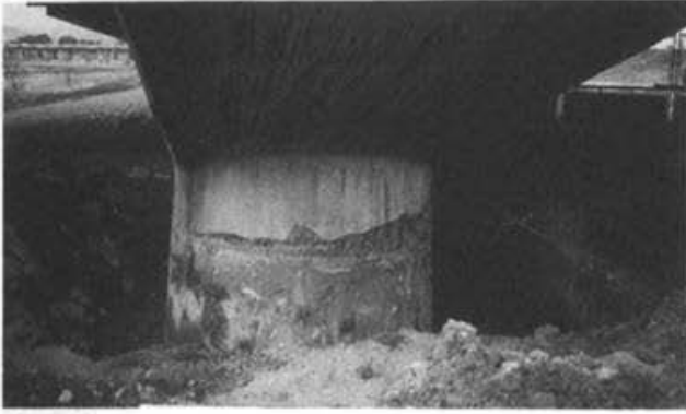
Photo 2.2.3 MEISHIN HIGHWAY (Mukogawa Bridge)
