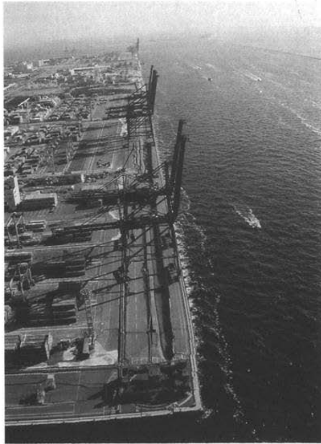
Figure 3 Damages of Seawall along South End of Rokko Island
