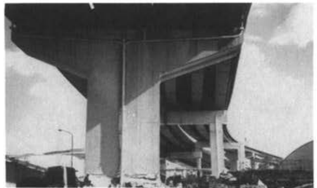
Photo 2.7.2 KOBE HARBOUR HIGHWAY
