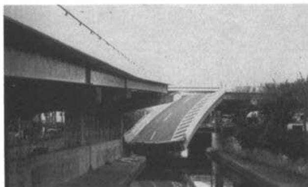
Photo 2.1.11 HANSHIN EXPRESSWAY (Minatogawa gate-way)
