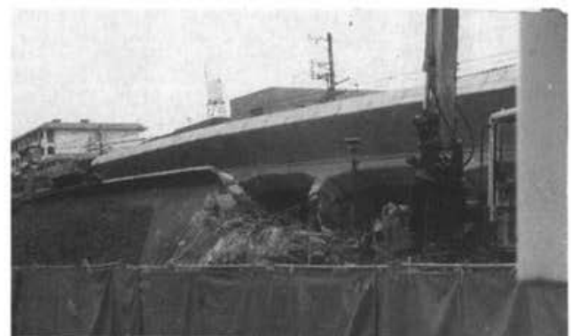
Photo 3.5.1 HANKYU LINE (Nishinomiya City - Murokawa-cho)
