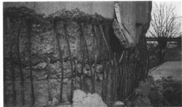
Photo 3.2.4 JR SHINKANSEN (Mukogawa Bridge)
