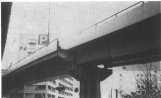
Photo 2.1.9 HANSHIN EXPRESSWAY (Chuo-Ward - Isogami-dori/ Ikutagawa Gateway)
