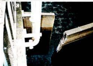
阻流壁破損
