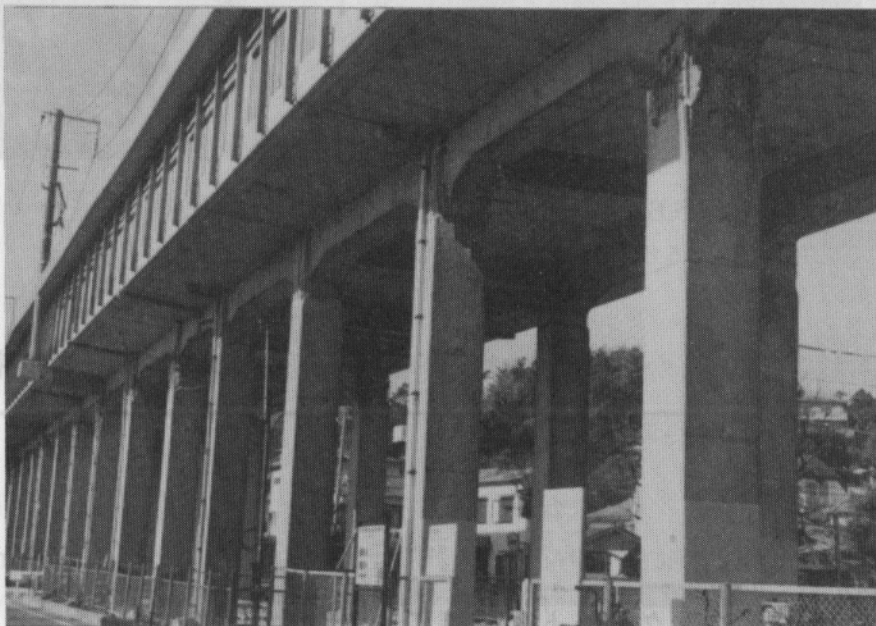
写真 5.6.2-10 橋脚頂部の破壊状況 Photo 5.6.2-10 Typical Frame Structure and Damage at Column Top
