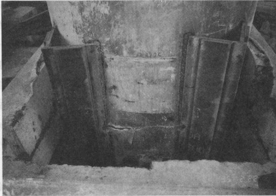
写真5.6.3-4 鋼製橋脚の根本全周脆性破断 Photo 5.6.3-4 Brittle Rupture of Steel Column
