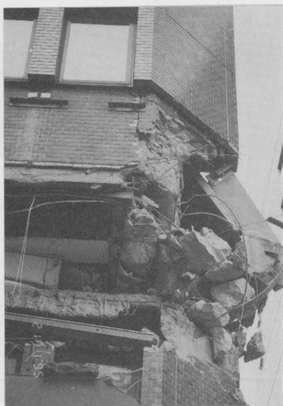
写真 5.2.1-7 SRC造の破壊状況 Photo. 5.2.1-7 Failures of SRC structure building
