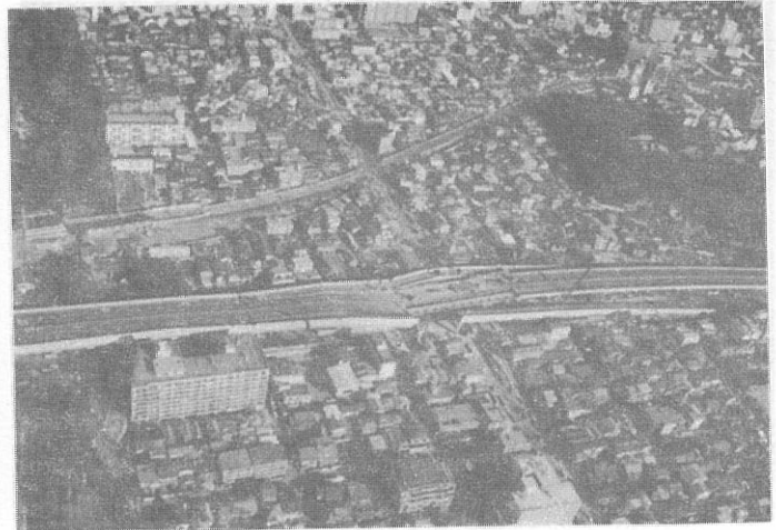
Photo 11 Collapse of a part of Hanshin expressway, Kobe route due to column failure
