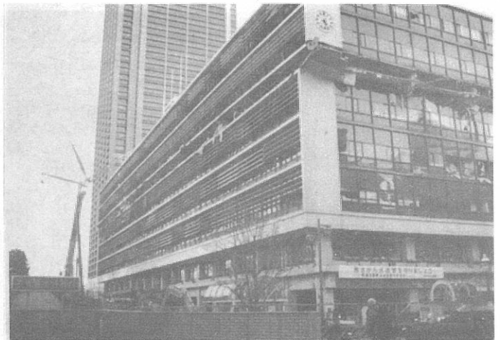
Photo 7 Collapse of the 6th floor of one of Kobe city hall buildings
