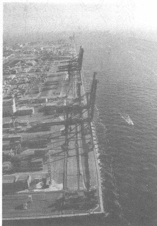
Photo 2 Damages to the seawall along south end of Rokko Island
