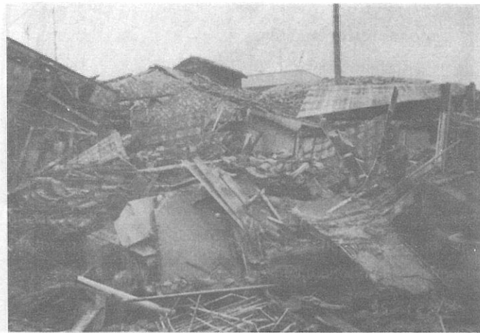
Photo 6 Total collapse of a timber house in Kobe
