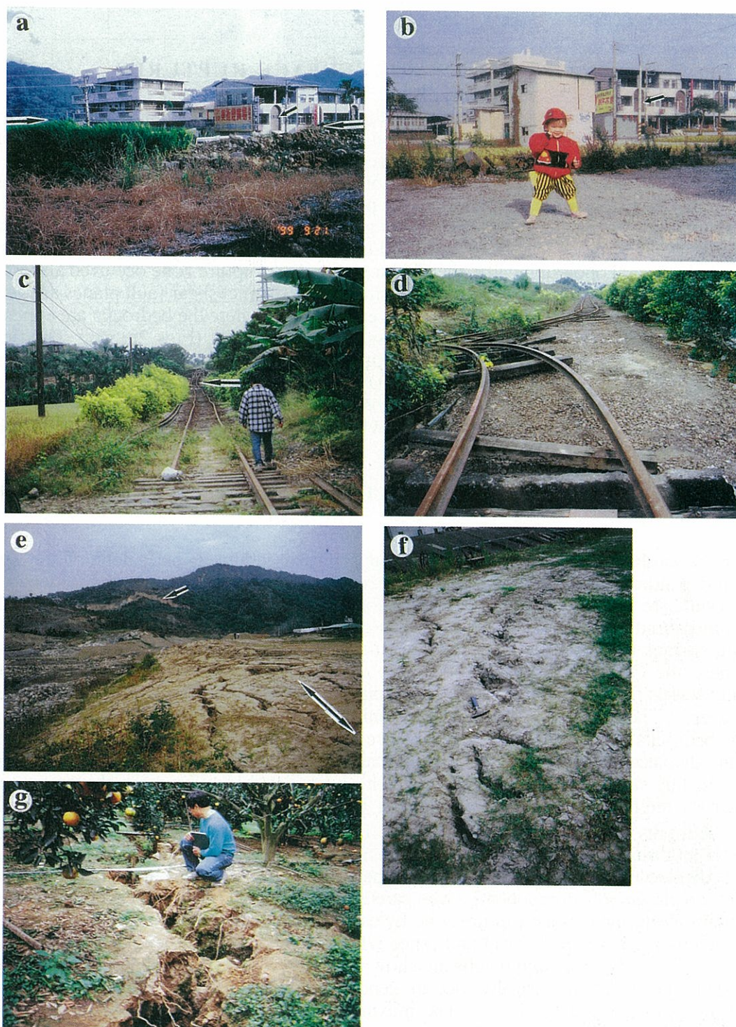
Fig.4. Deformational topographies generated by the co-seismic faulting. (a) and (b): The change in topography occurred at Loc.4 before (b) and after (a) the earthquake. Large arrows indicate the flexure-fault scarp. Note that the first floor of the building was in sight of the photo before the earthquake (b) but is out of sight in the photo (a). Small arrows indicate the same window of the building shown in (a) and (b). Both photos were taken from the same location and view direction by the landlord (Mr. Z.Z. Sheng) (view northwest). This indicates that the east side was uplift one-floor high during the earthquake. (c) and (d): The railway was bent by the co-seismic faulting and folding at Loc.12 near the epicenter Chi-Chi town. Arrow indicates the fault scarp in (c) where the railway was sinistrally displaced about 1.7 m (view east). (e): Extensional cracks occurred at Loc.10 in the hinge area of the flexure-folding structures (view east). The large arrows indicate the strike of the hinge line. Note that the large-scale landslide (indicated by the small arrow) occurred near the surface rupture zone. (f): Extensional cracks show a Left-step en echelon form occurred at Loc.4 (view east). (g) Extensional cracks occurred in the jog area between two distinct shear faults at Loc.2 (view southeast).
