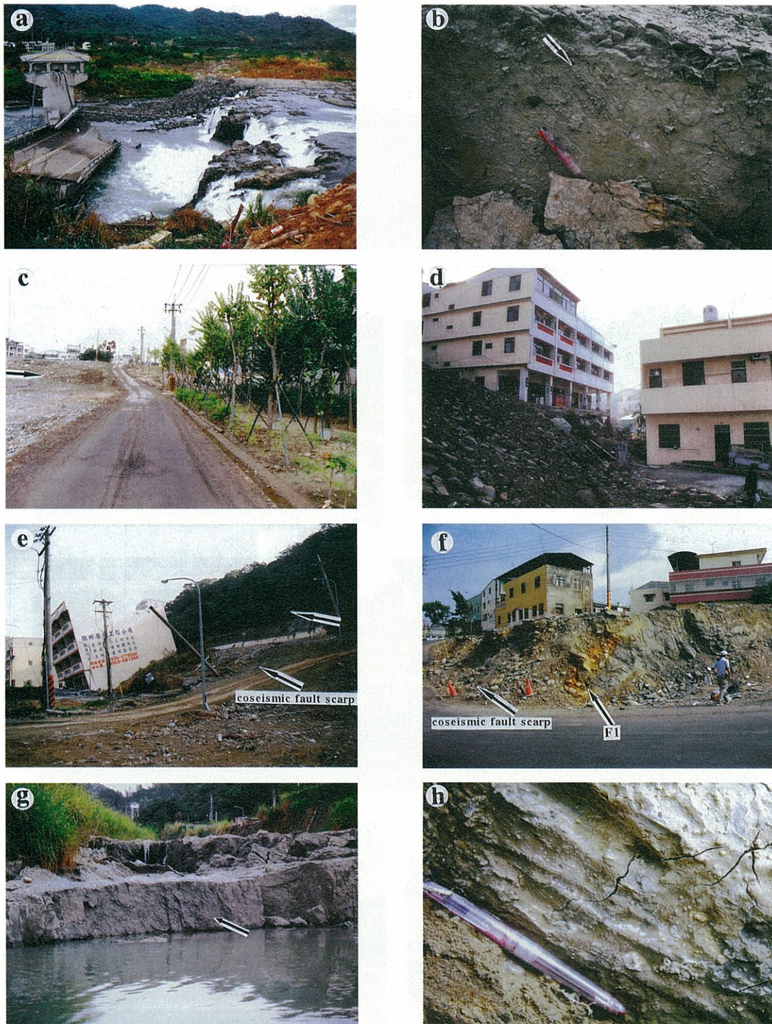
Fig.2. Typical fault outcrops of the Chelungpu surface rupture zone. (a): The river channel at Loc.3 (shown in Fig.7) was displaced and uplift about 6.7 m in the hanging wall (view northeast). (b): Striations generated by the co-seismic displacement on the fault plane at the Loc.3. Arrow indicates the slip direction of the lost wall. (c): The road was sinistraly displaced about 7.0 m at Loc.4 (view northwest). Arrow indicates the co-seismic fault scarp. (d): Fault scarp occurred in terrace deposits at Loc.7. Note that the buildings on both sides near the fault scarp were only gently damaged (view southeast). (e): The co-seismic fault scarp at the location near Loc.7 occurred along the pre-existing fault scarp (indicated by arrows on the upper side) (view east). Note that the building was tilted and damaged by faulting on the fault scarp (view northeast). (f): Co-seismic fault scarp occurred in a pre-existing fault zone at Loc.8. F1 is a pre-existing fault plane, where the overlain terrace deposits are not deformed or displaced by the co-seismic faulting during the Chi-Chi earthquake (view southeast). (g): Fault scarp occurred in the bedrock at Loc.8. Striations (indicated by arrows) can be observed on the fault plane (view east). (h): Grooves and striations generated on the fault plane shown in (g).
