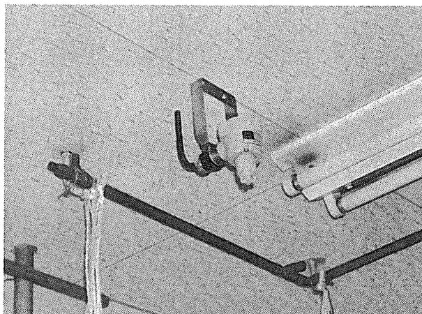
Fig.3-1 Picture of a hydrogen gas sensor.
