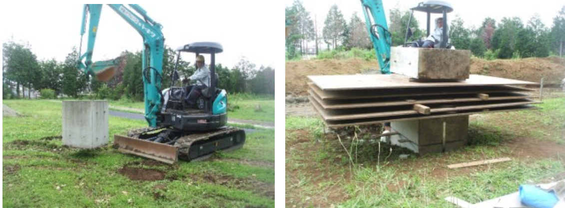
Fig. 2-10 上载荷重の負荷状況 Appearance of upper load
