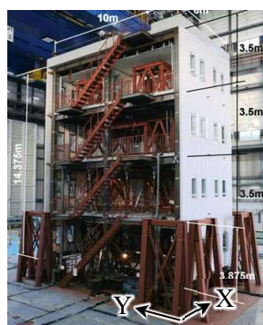
(a) Four-story steel structure building (S4)
