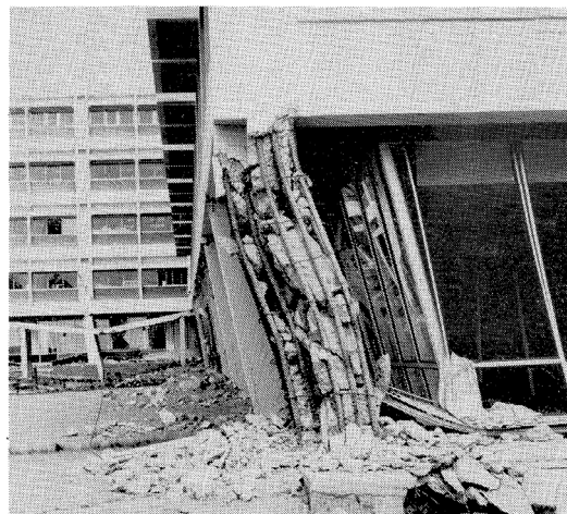
FIG. 3.10 DAMAGE TO FIRST STORY COLUMN BB-3 ILLUSTRATING SEVERITY OF FIRST STORY DRIFTS AND SUBSIDENCE OF NORTHERN TERRACE CANOPY DUE TO FAILURE OF COLUMNS IN CRAWL SPACE
