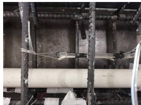
(b) Install in reinforcement cage
