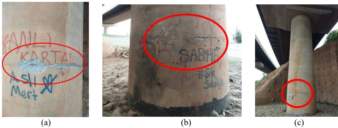
Figure 8 Different views of plastic hinge formation
