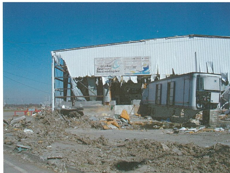
Photo #33. Biloxi, MS. Fishing industry warehouse destroyed by the surge.
