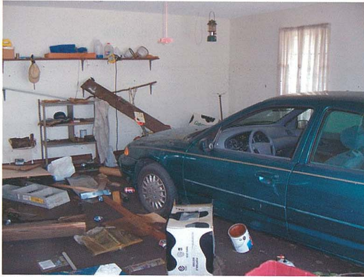
Photo #40. Slidell, LA. Debris line in this garage indicates the maximum flood level. Photo courtesy Kirk Thibodeaux.
