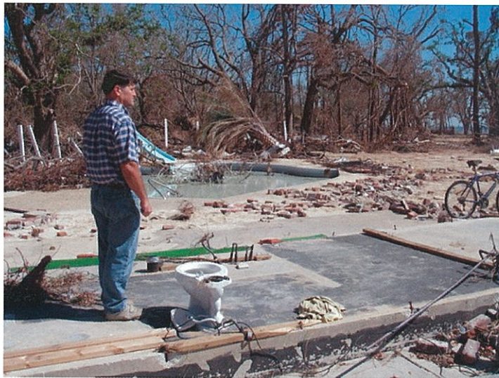
Photo #10. Waveland, MS. Brick home destroyed by the surge. Only the toilet was left standing.
