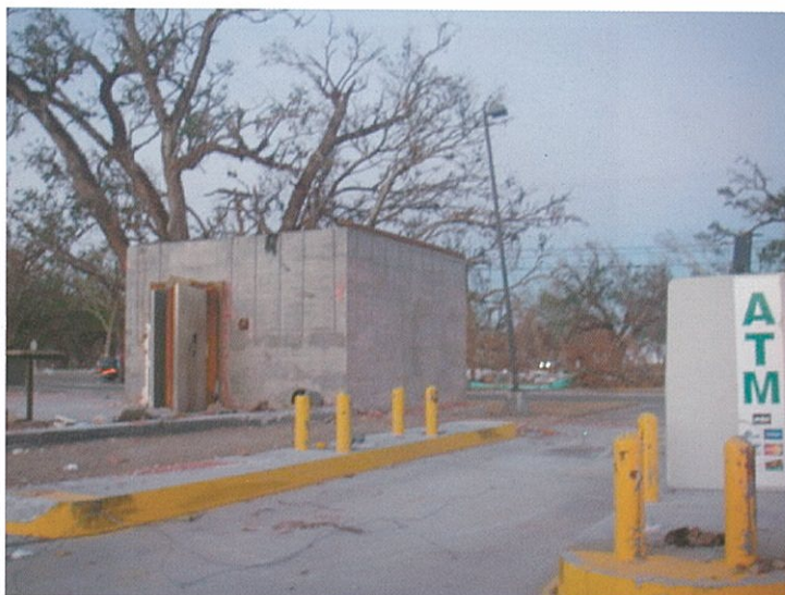
Photo #24. Pass Christian, MS. Vault of a bank. The rest of the building was destroyed in the surge.
