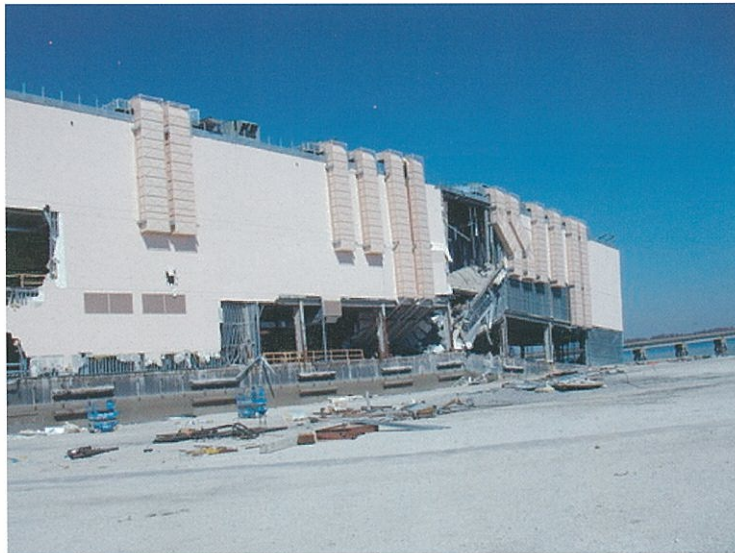
Photo #37. Biloxi, MS. Casino barge deposited in a parking lot.
