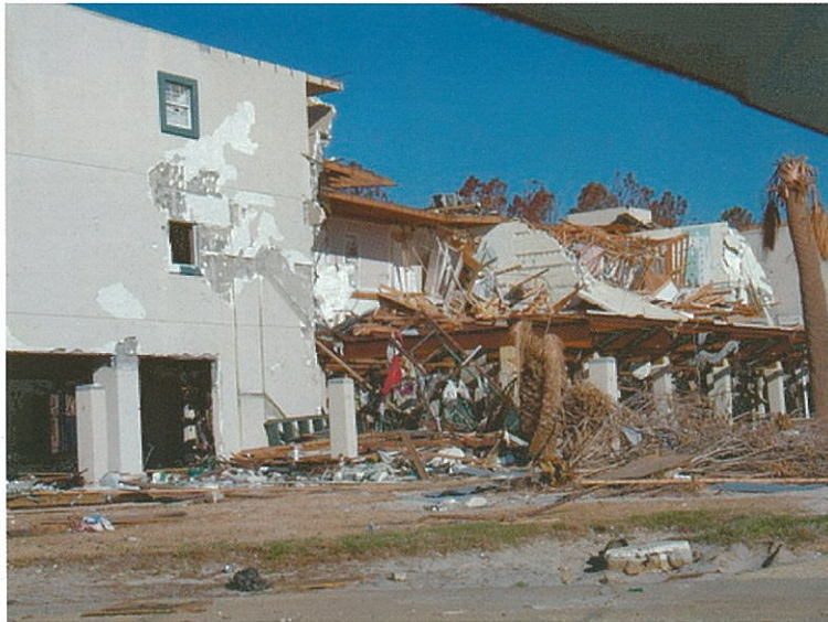
Photo #31. Pass Christian, MS. Wrecked building near the beach.
