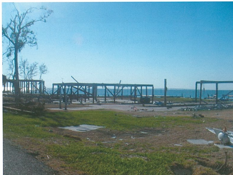
Photo #44. Rigolets, LA. Piles on which sat homes that the surge carried away.
