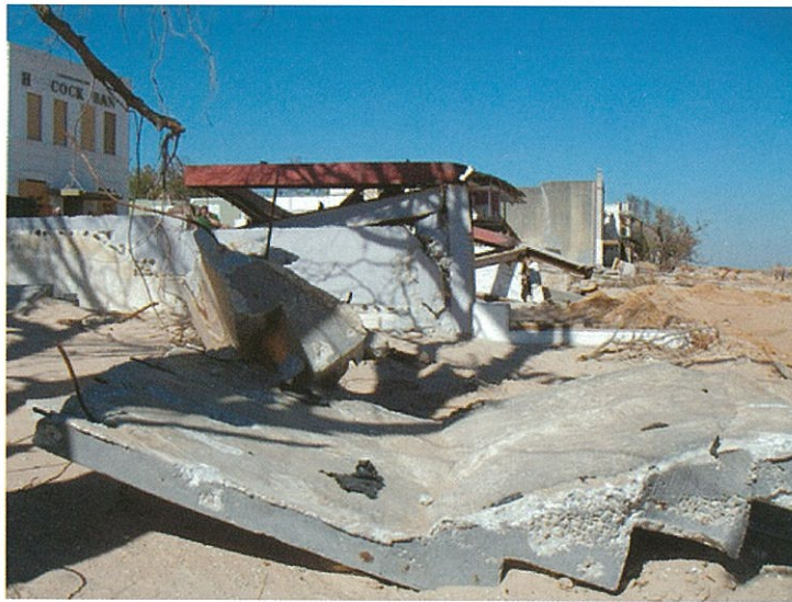
Photo #16. Bay St. Louis, MS. Steel-frame and reinforced-concrete restaurant on the beach, destroyed by the surge.
