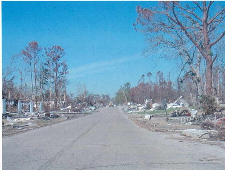
Photo #8. Waveland, MS. Restaurants, shops, and homes devastated by the surge.
