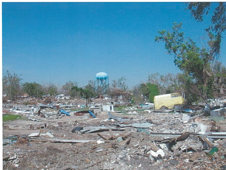
Photo #39. Biloxi, MS. Typical scene of the destruction caused by the surge in residential areas.
