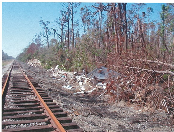
Photo #12. Waveland, MS. Railroad ballast scoured seaward by the surge, along with large, buoyant debris which had been advected landward by the surge and then deposited on the seaward side of the railroad.
