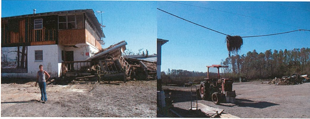
Photo #1. Pearlington, MS. Restaurant damaged by the surge (left) and marsh grass deposited by the surge on telephone lines (right).
