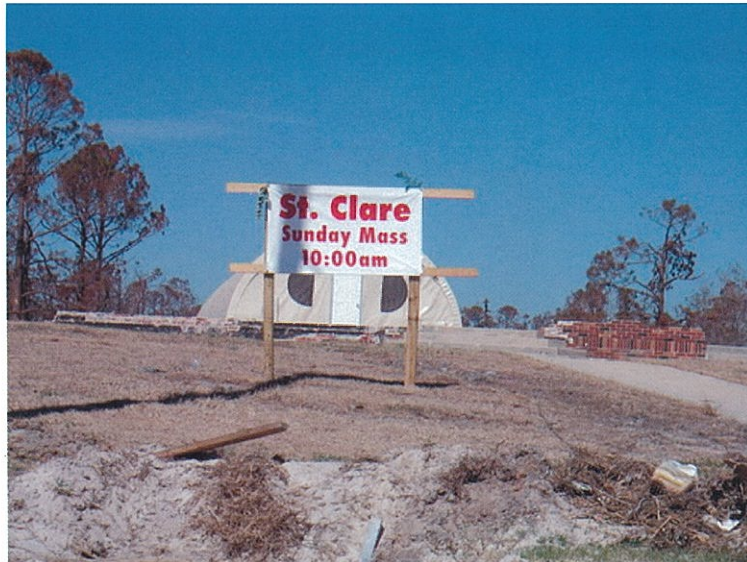
Photo #7. Waveland, MS. Tent sitting on the foundation of a wrecked brick church.
