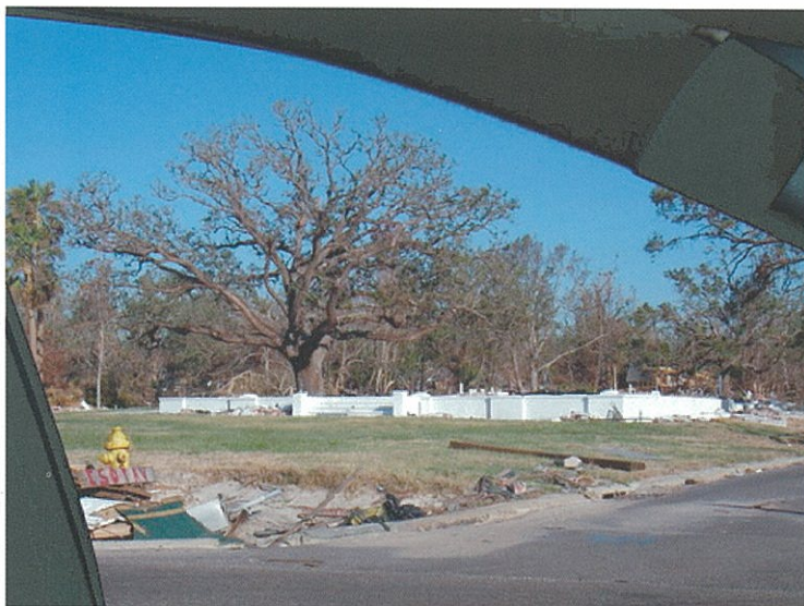
Photo #30. Pass Christian, MS. Home and road were destroyed, but foundation and fire hydrant remain.
