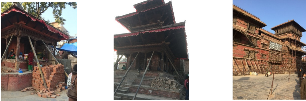
Photo. 1. Two temples and Durbar Square in Basantapur area under temporary supports (Photo taken on Feb. 2017)
