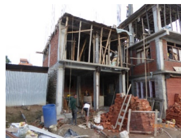
Photo. 5. New buildings on private funding coming up (Sept, 2016)
