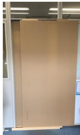
Figure 3: Outlook of the mockup plenum structure set in an opening in the partition between the offices used for the experiments.
