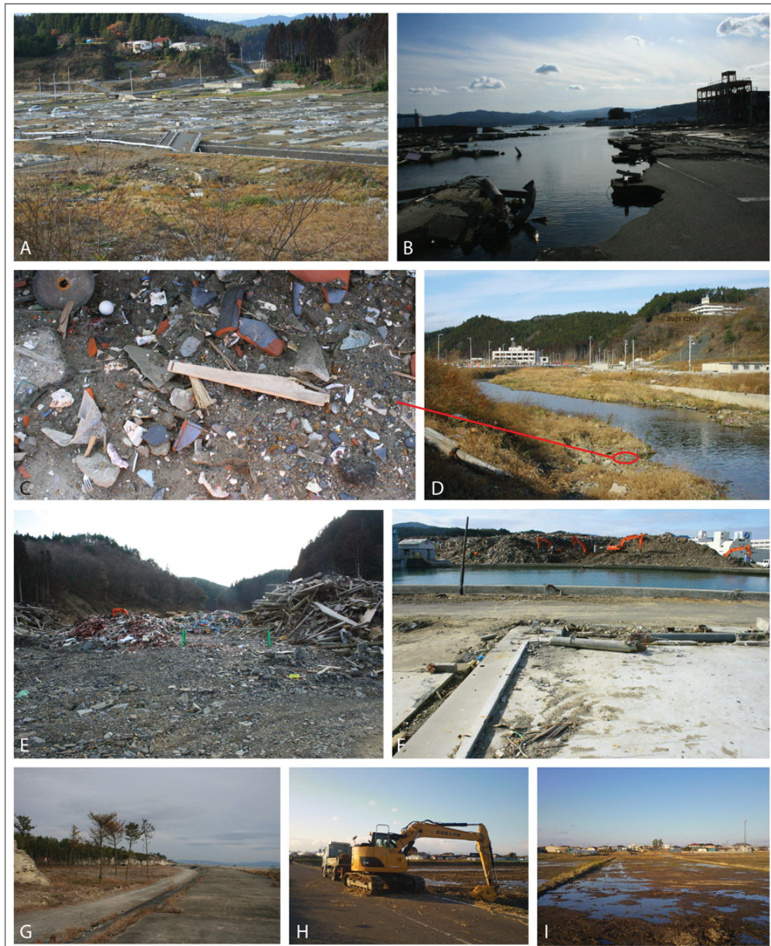
Figure 12. The Tohoku tsunami in 2011 (Japan) and its interaction with anthropogenic environments: (A) House slabs and collapsed bridge in Kesenuma; (B) The eroded and undermined Minami-Sanriku port area infrastructure; (C and D) Tsunami backwash deposits in a Minami-Sanriku riverbed; (E) Material near Motoyoshi in a valley near the train-line; (F) Debris being gathered and transported away in Minami-Sanriku; (G) Coastline in Higashi-Matushima; (H) Excavation of sandy sediments from Sendai plain rice fields; (I) Excavated Sendai rice field.
