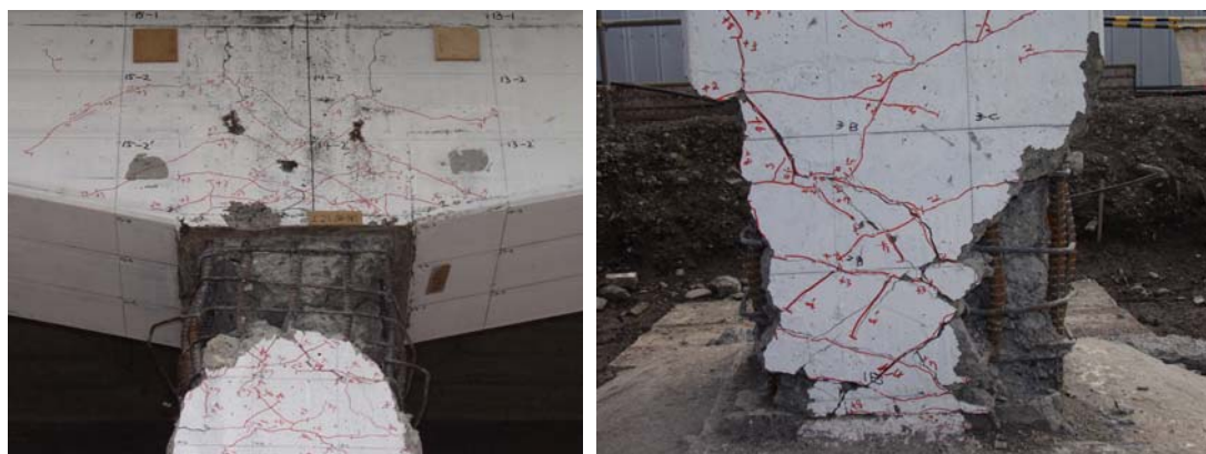
(a) Top of a column (No.2L)
