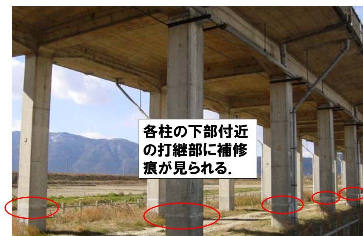
Fig.3-14 Condition of columns of viaduct-G
