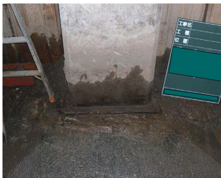
Fig.3-15 Condition of column and footing of viaduct- H
