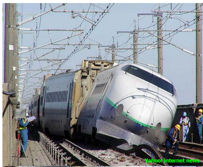
Derailment accident in Niigata earthquake
