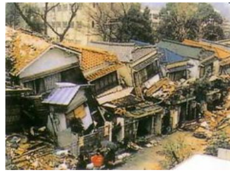
Damage for Residential Buildings
