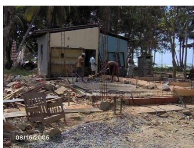
Reconstruction of a partially damage house
