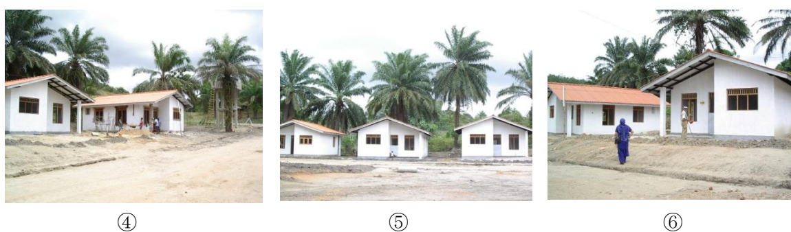
Fig.3.15: Walahanduwa- Salsberg Village Permanent Housing Settlement at Under Construction Stage on 2005
