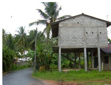
Completed house up to structural level-2007
