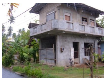
Completed house up to basic finishes level-2008
