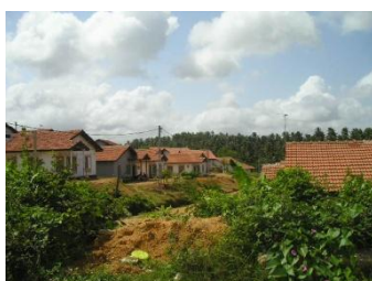
⑤ Inside view of the settlement-2006
