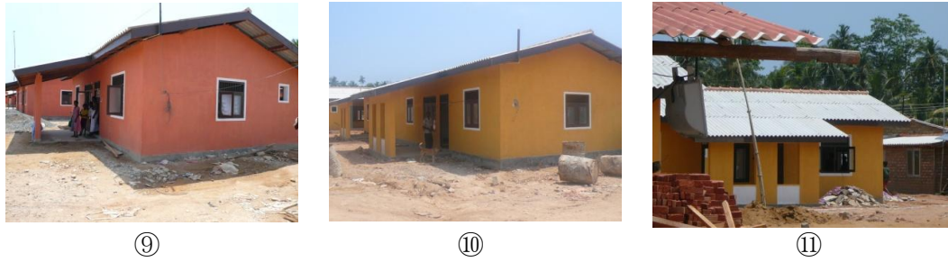
Fig.3.36: Mirihanawatta Permanent Housing Scheme – under construction 2007
