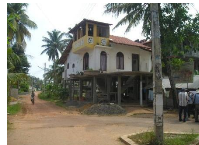
Completed house up to finishes level-2007
