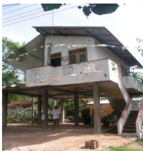
Completed house up to basic finishes level-2007
