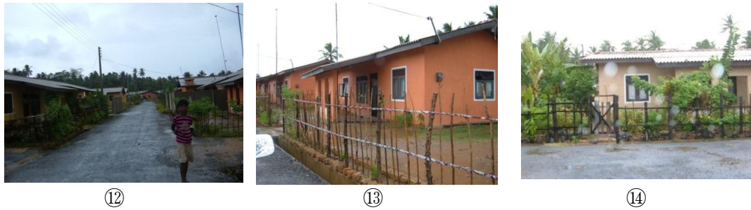
View after completion of roads In side views of the well established settlement -2008
