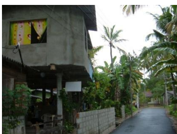
Completed house up to basic finishes level-2008
