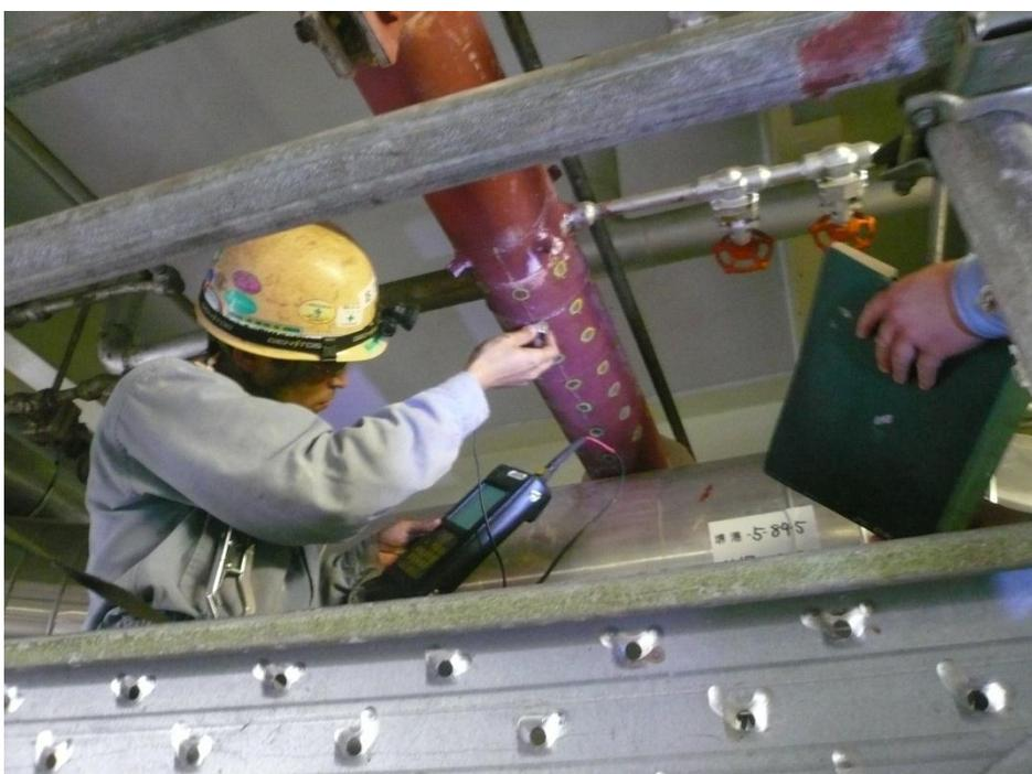
**Fig. 1.2.1-6: Thickness measurement work using UT. Measurements are performed by two workers. Main worker measures wall thickness. Another worker records measurement results.**
