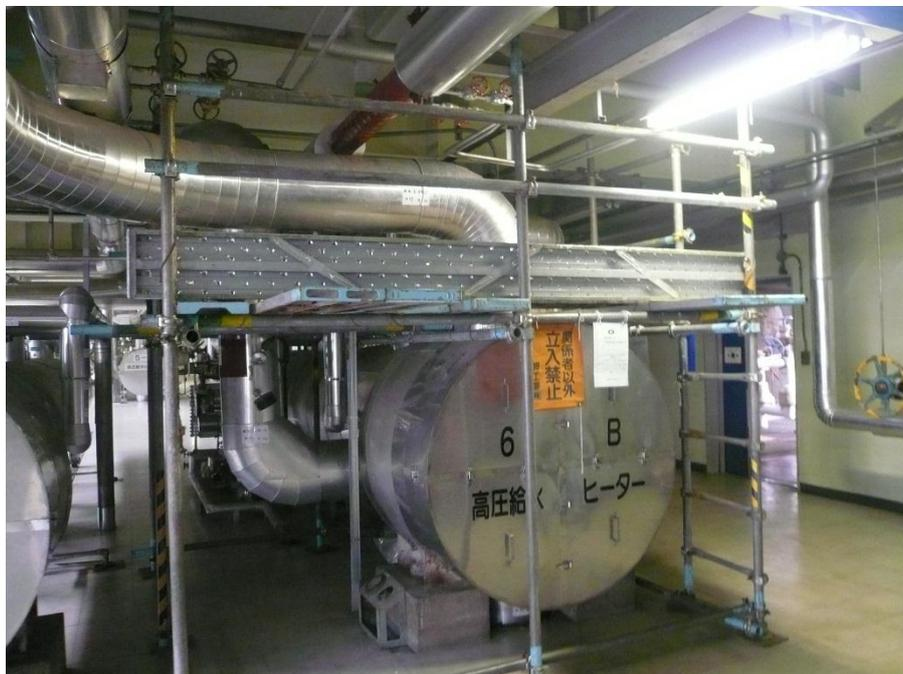
Fig. 1.2.1-4: Scaffolding for thickness measurement. Scaffolding must be made, when work location is a high place.
