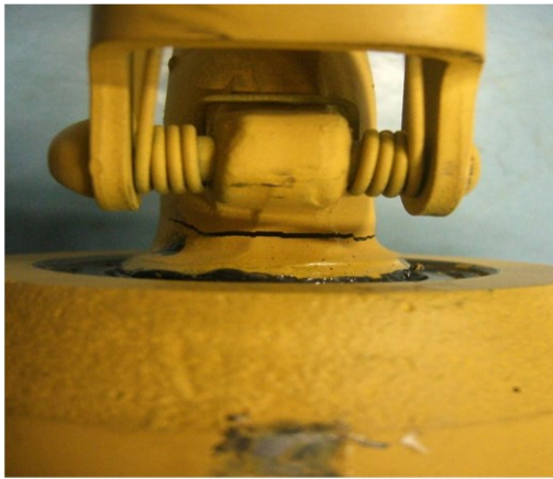
1) with grease (3.6 ton)
