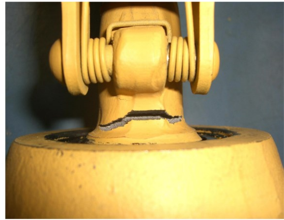
2) without grease (3.6 ton)
