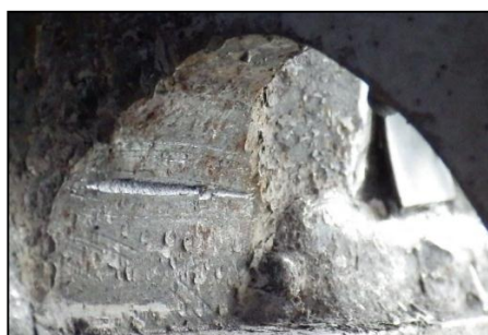
(c) CBS-29: Crack initiation
