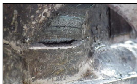
(b) CB-29: Crack progress(width:0.9mm)
