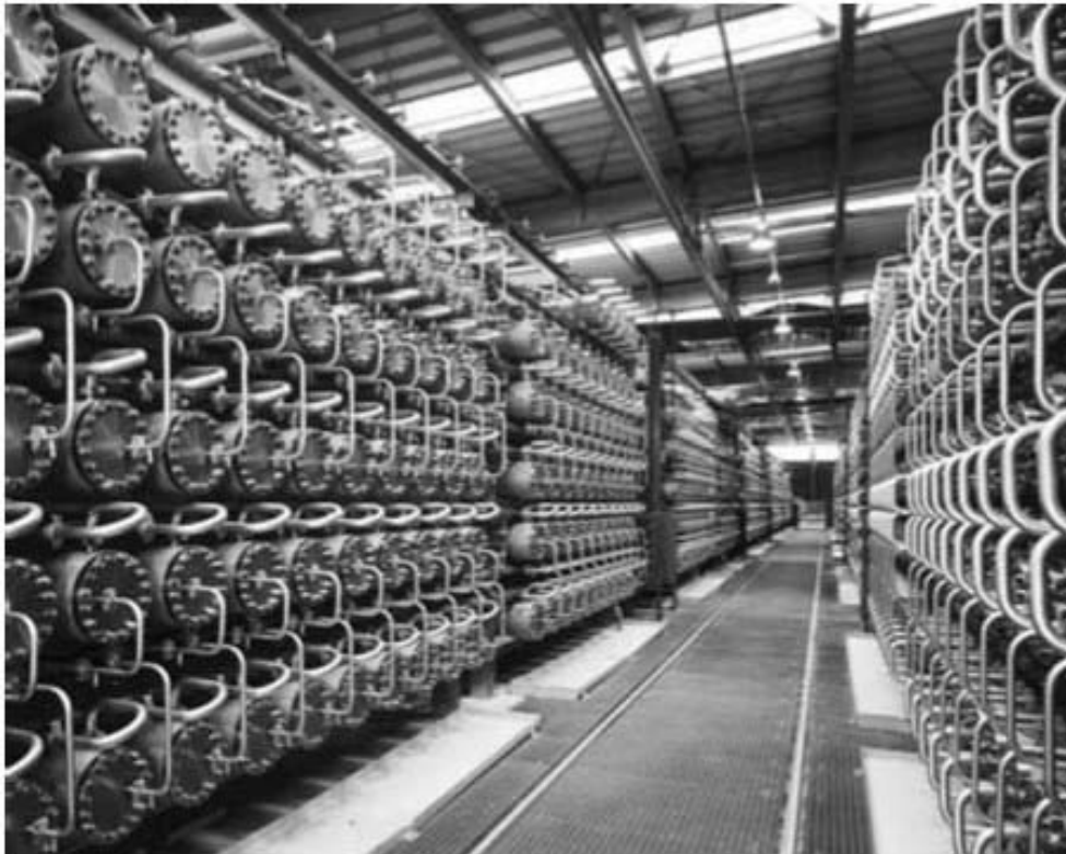
Fig. 1.5. Recent high-pressure RO module unit [6]
