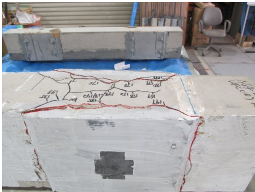
(a) Bottom of beam
