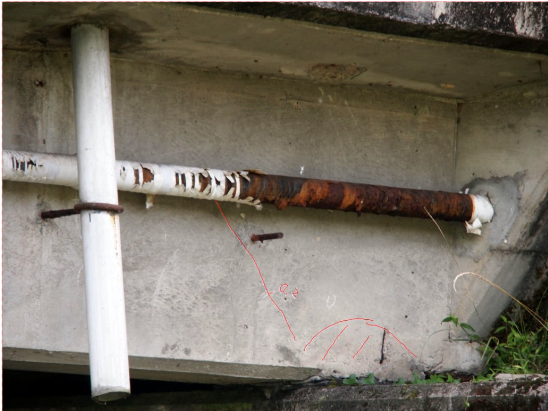
Fig. 1.1. Girder end of an aging bridge built in 1960s in Japan.
