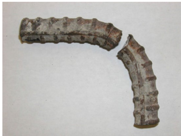
Fig. 5.1. Fracture of tensile rebar anchor
