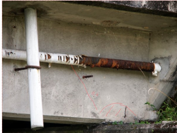
Fig. 6.1. Girder end of an aging bridge built in 1960s in Japan.
