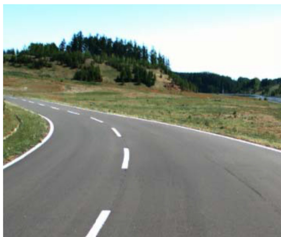
Fig.3.2: The road where curvature changes
