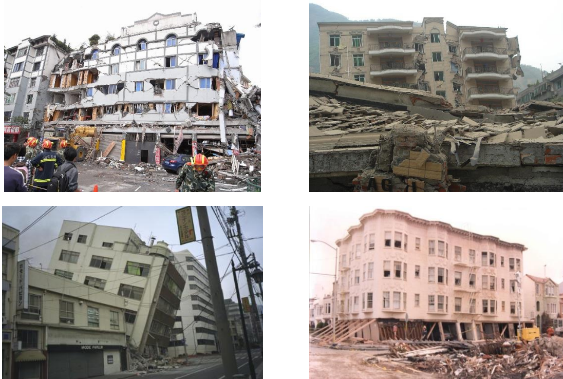
Fig.1 - 2 Damaged concrete buildings in earthquake[1.14-1.17]
