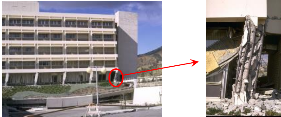
Fig.3- 1 Damage to the Olive View Hospital in the 1971 San Fernando earthquake (Steinbrugge K. V., NISEE Database) [3-2]
