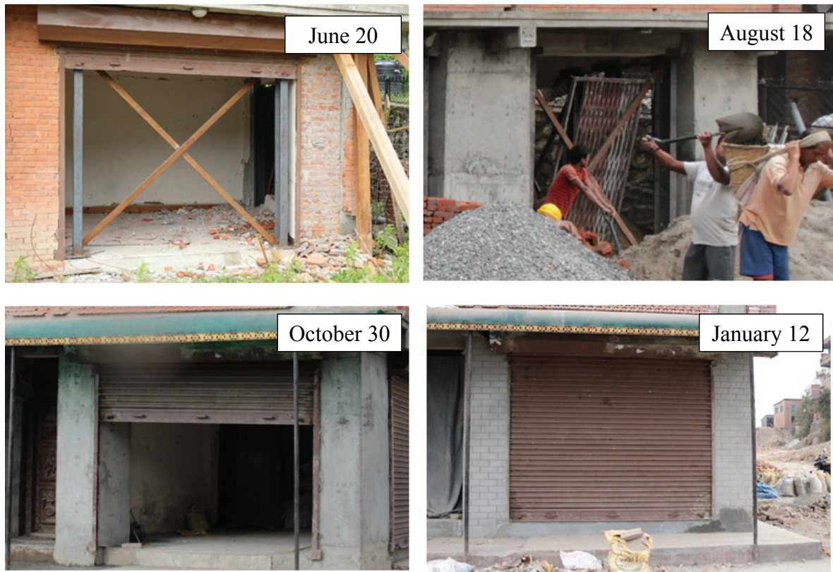
Figure 9 Progress of earthquake repairs on a cracked corner
