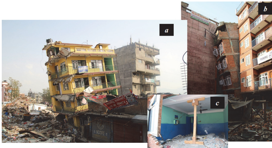
Figure 17 At Gongabu, RC frame buildings were tilted ( a,b ). A shear crack in the first floor ( c )
