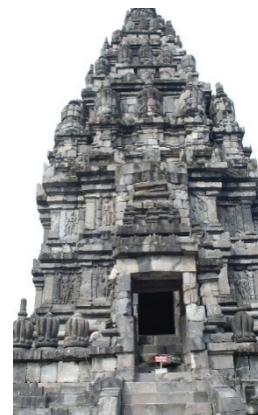
Figure 15 The Wisnu temple sustained relatively little damage.
