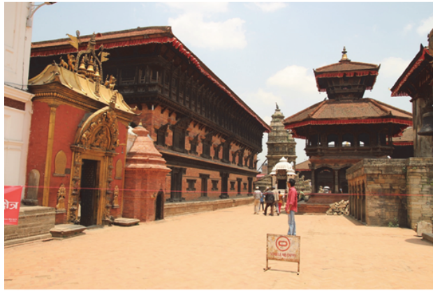
After the earthquake
