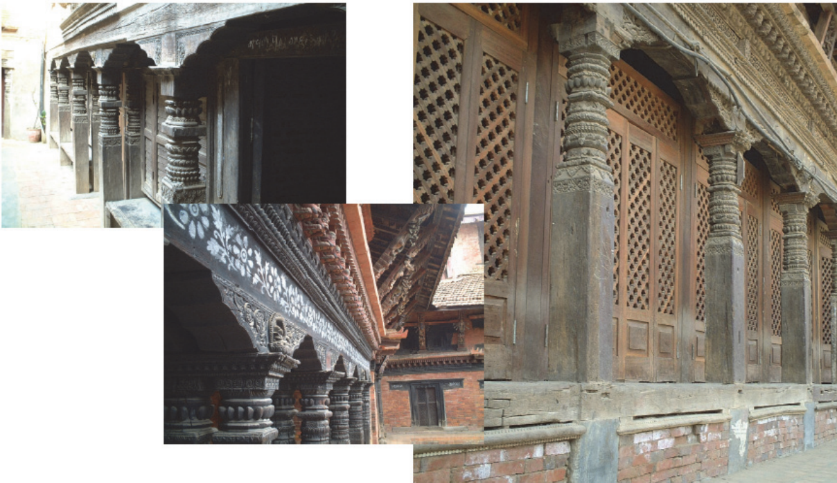
Figure 8 Peristyle colonnade in Patan (photo by T.Ohsumi after the 2015 Earthquake).
