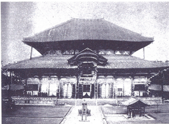
Figure 3 The lower roof fell down to the Todai-ji Temple Great Buddha hall in the Meiji era.
