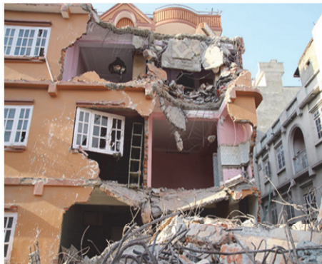
Figure 18 At the branch point of the Bagmati River and the Transformer River, collapsed building fell onto and destroyed the next building (photo by T. Ohsumi).
