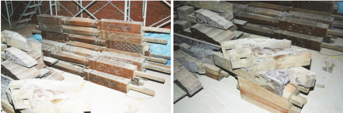
Figure 6 Columns and sub-beams (parts of the replica temple with EXPO 2005 AICHI JAPAN: photo by T. Ohsumi in 2005).
