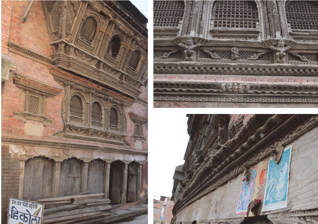
Figure 17 Masonry building with a Naga band installed that survived the 2015 Gorkha Earthquake in Sankhu (photo by T. Ohsumi after the 2015 Earthquake).
