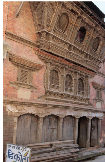
Figure 2 Masonry building with a Naga pasa .
