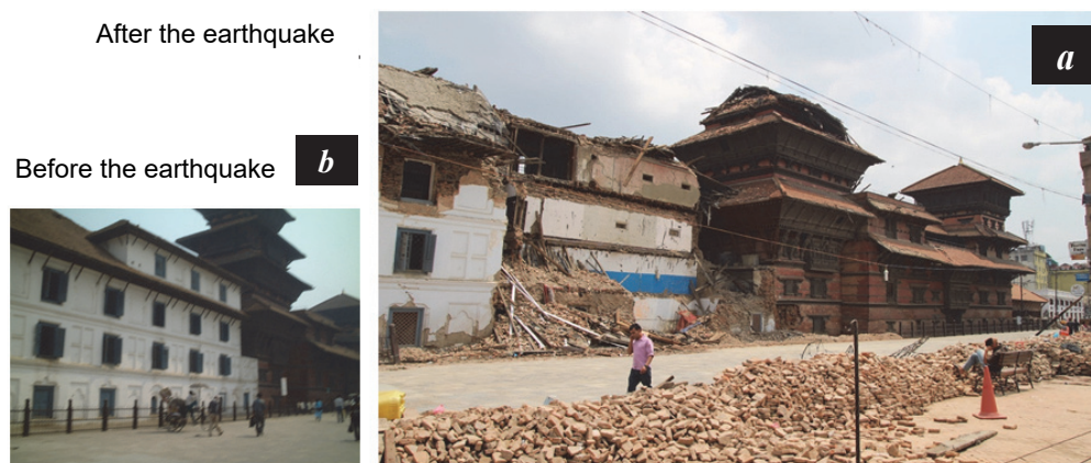
Figure 16 Kathmandu Durbar Square after the earthquake ( a ), before the earthquake ( b )
