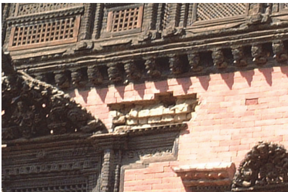
Figure 25 Scree of bricks. Sun-dried bricks (adobe) of the interior are seen (photo by T. Ohsumi in 2001).
