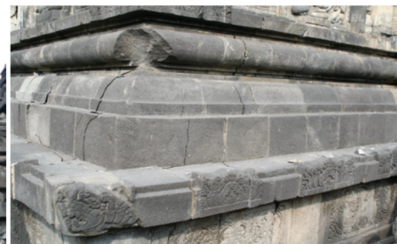
Figure 13 The gallery of the Siwa temple were damaged. Some cracks appeared in the corner section of this temple. All corner sections of the Siwa temple had cracks.
