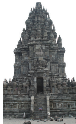
Figure 14 All corner sections of the Siwa temple had cracks.
