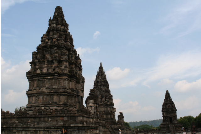
Figure 19 The damage sustained was not so serious at the Nandi temple ( right ) and the Angsa temple ( center ). (photo by T. Ohsumi)
