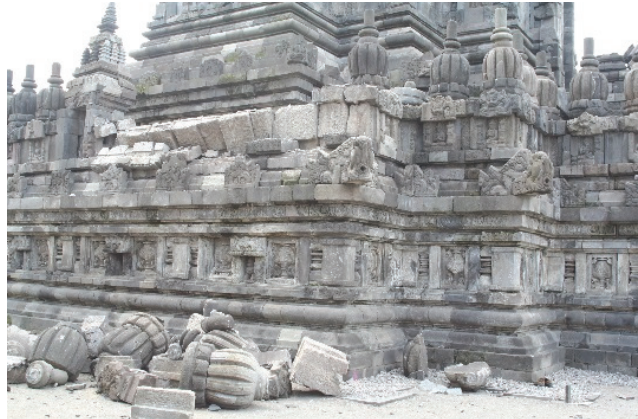
Figure 18 The Garuda temple is leaning due to the earthquake. (photo by T. Ohsumi)
