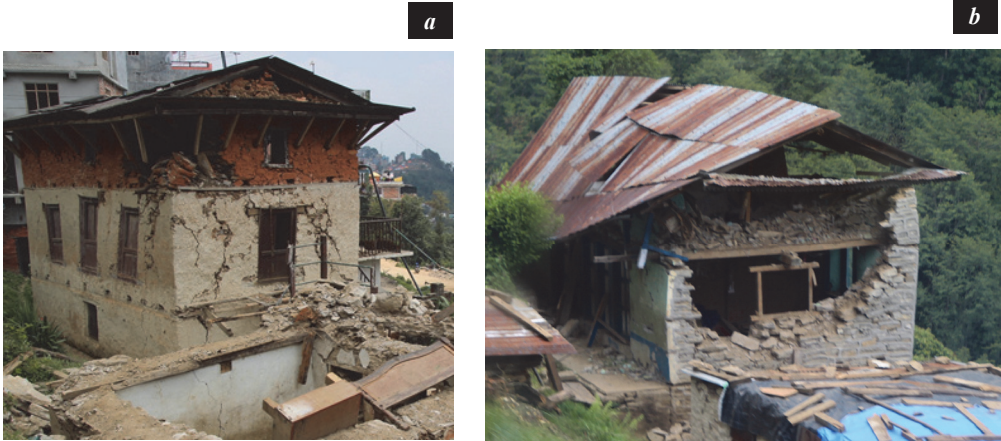
Figure 5 Adobe style houses (a) and Stone style house (b) in Charikot, (photo by T. Ohsumi)
