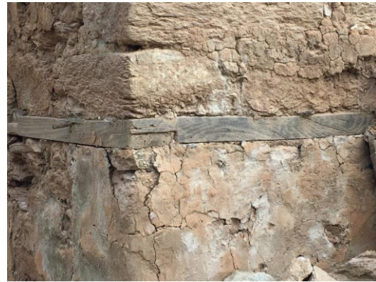
Figure 5 Corner joint of horizontal timber planks
