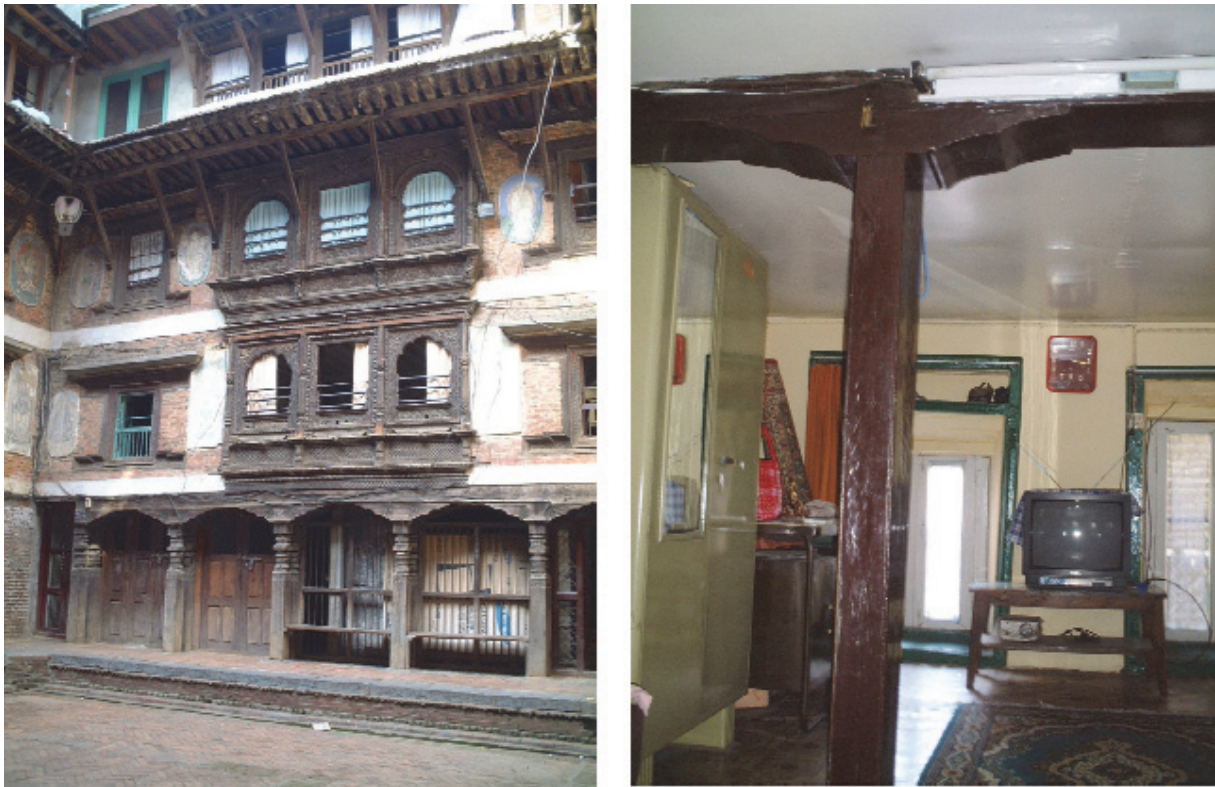
Figure 9 House's peristyle colonnade and indoor column with a sub-beam in Patan (photo by T. Ohsumi in 2001).
