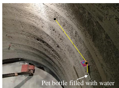
Figure 3.17 Monitoring of the change in length of the arch section (No.1375R)
