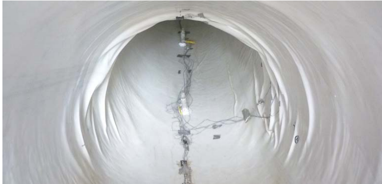
Figure 4.5 Wrinkles at the bend.
