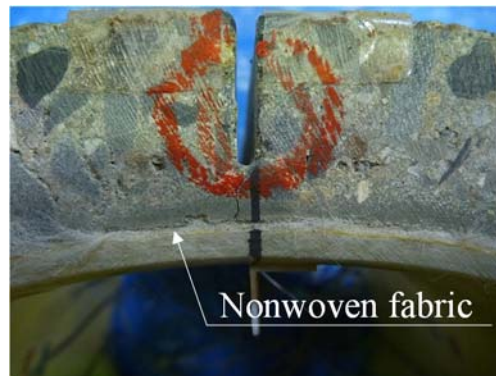
Figure 5.4 Non-woven fabric between existing pipe and liner.
