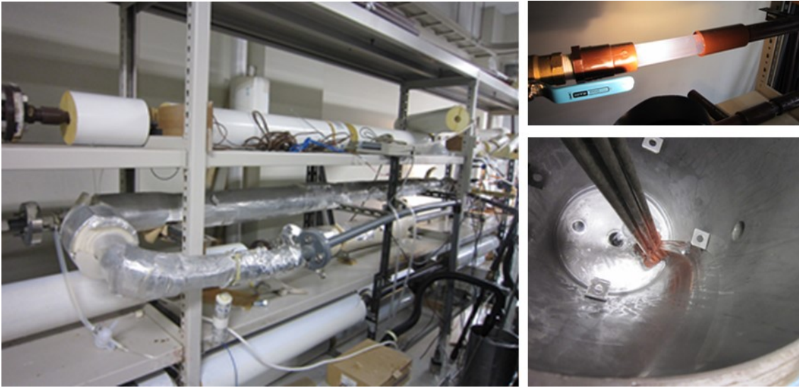
Fig. 3-4 Pictures of the pipe flow systems with double pipe heat exchangers
