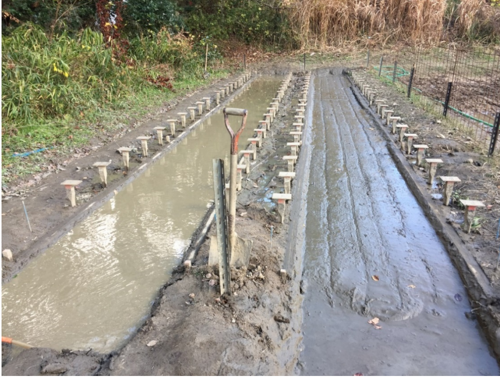
Figure 2.3 The testing field with uniform soil pan: in the left, hardpan 11 cm filled with water and in the right, hardpan 16 cm before flooding.
