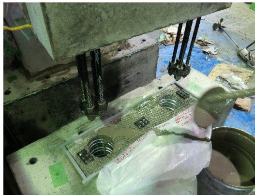
Fig. 3.2-1 Assembly of the precast wall
