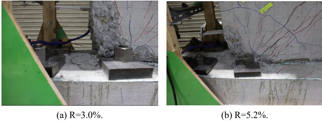
Fig. 4.3-2 Damage observed on specimen WP15-D10H55P-075
