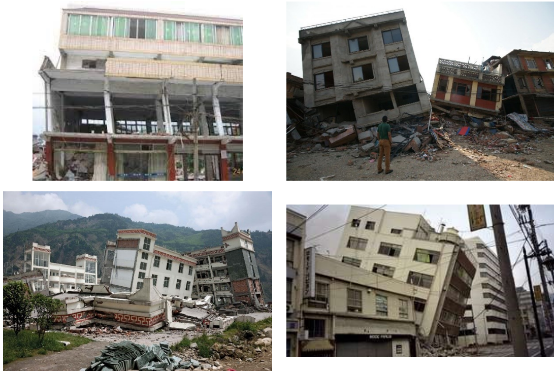
Fig. 1.1-1 Damaged ductile concrete building in major earthquakes [1.16-1.19]
