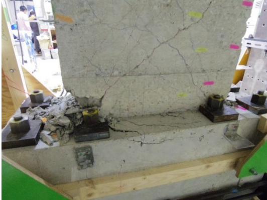
Fig. 2.3-8 Damage at beam-wall joint (specimen W15-HU-073 at the loading cycle of 4%.)
