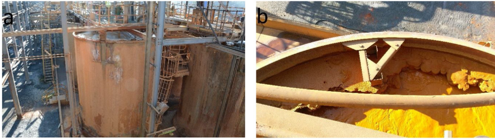
Figure 1.3: Example of scale formation in a mineral processing plant (a) neutralisation tank, (b) scale grown on its walls, from the paper by Davoody et al. 63
