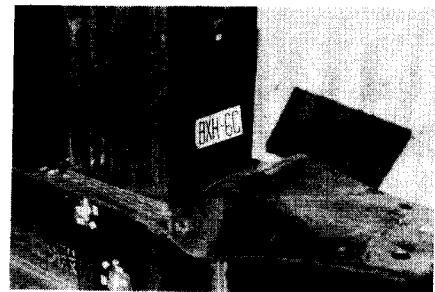
Photo 4.2 Local buckling of diaphragm
